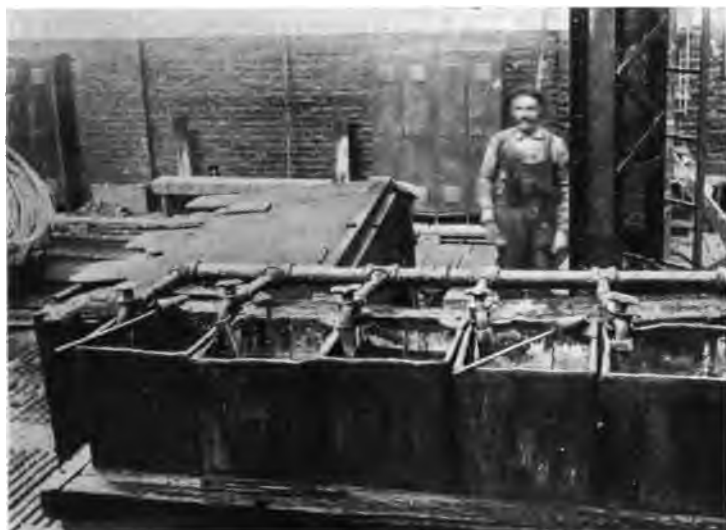
Fig. 3. Safety Acid Handling System in Wire Mill Cleaning House.*
